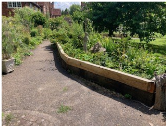
G: H: & J: Illustrating banks which were created from the earth removed when making the new pathway. By creating the banks the level of the plants is higher and brings them into closer to the field of visitors especially those in wheelchairs
